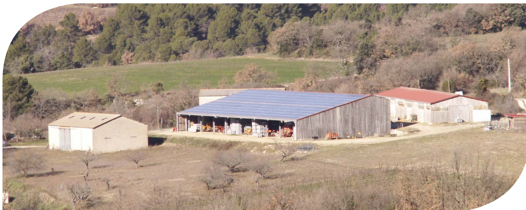
● Hangar photovoltaïque – Caseneuve [84]
